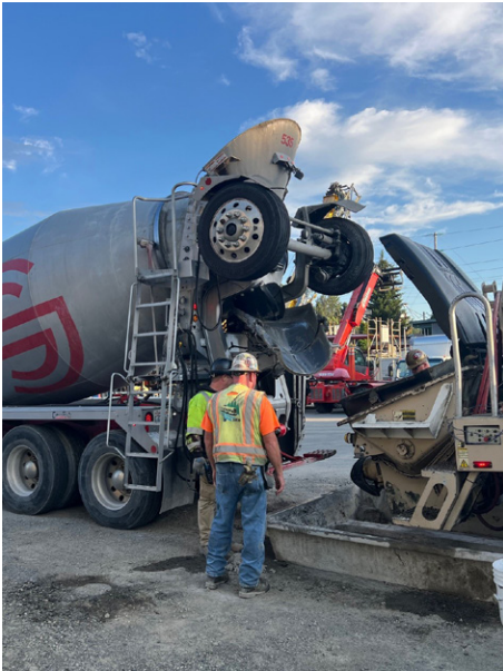
Testing of Truck Trial Mixtures
