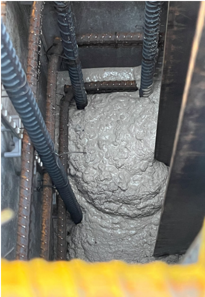
Testing, Placement, and Final Column Encasement for Pumped Column Concrete
